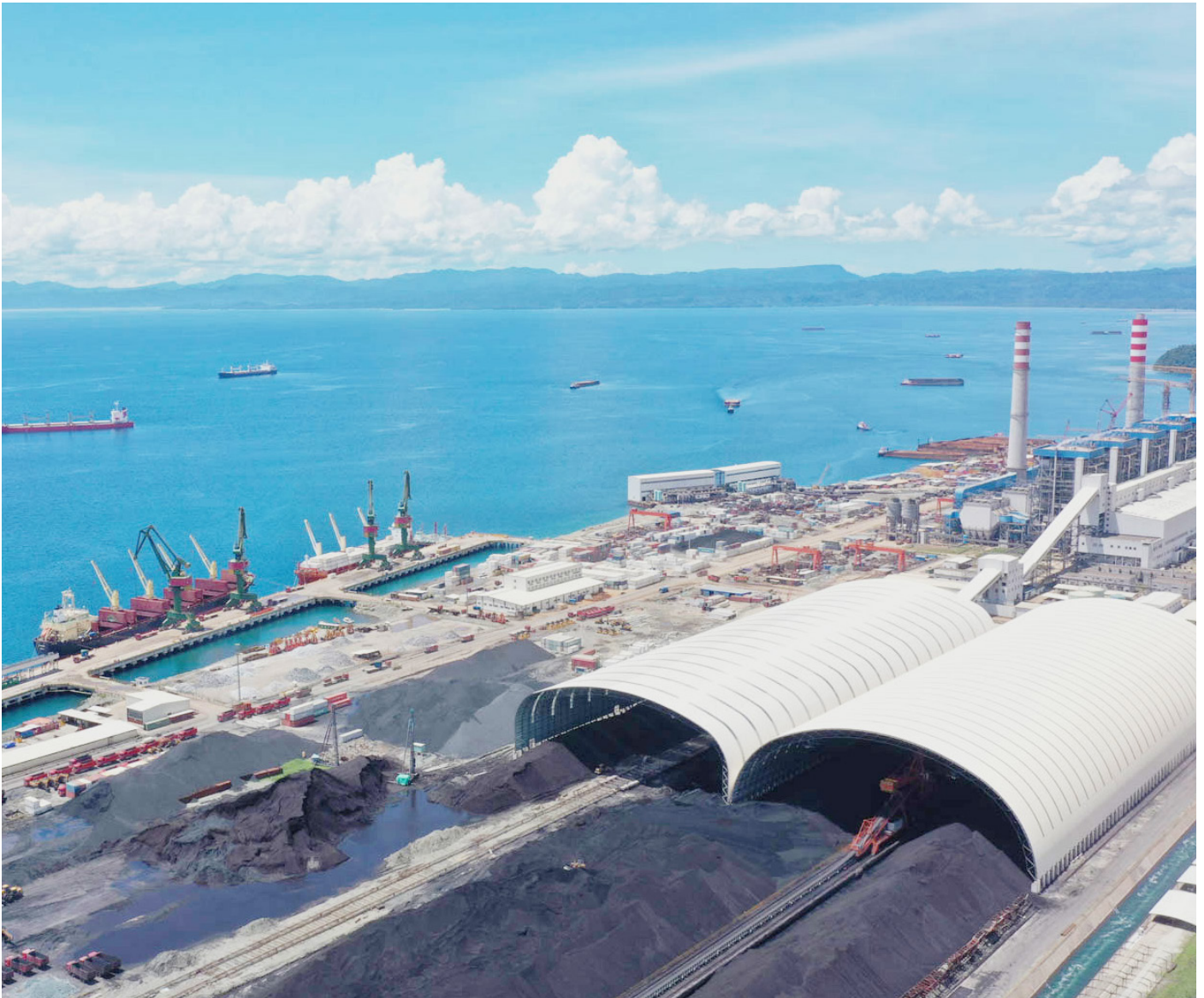
Indonesia Weda Bay Industrial Park in construction
