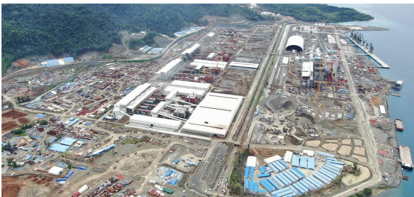
Indonesia Weda Bay Industrial Park in construction
